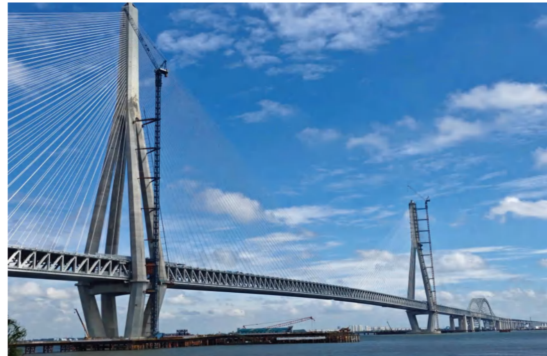
常泰大桥 CHANGTAI BRIDGE
