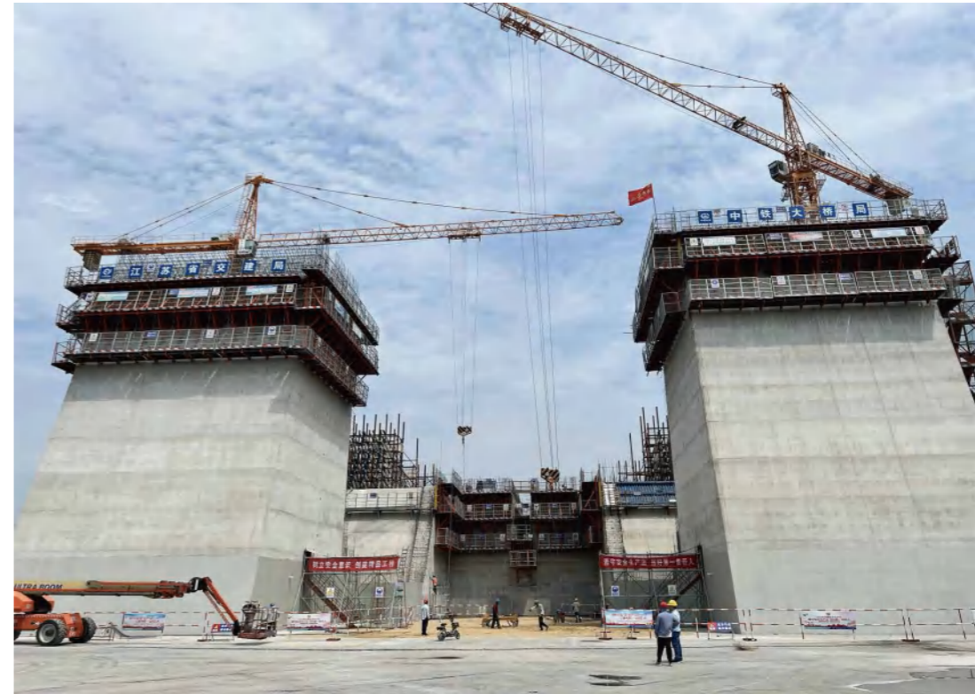
龙潭大桥 YONGLONGTAN BRIDGE
